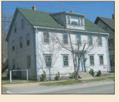
windows over four windows with the door below the center window and the clapboard siding all typify early heritage homes. Of interest is the old style in which the new clapboard has been applied. It tapers at the bottom to protect the sills from water damage. Reproduction "rose head" nails have also been used for
